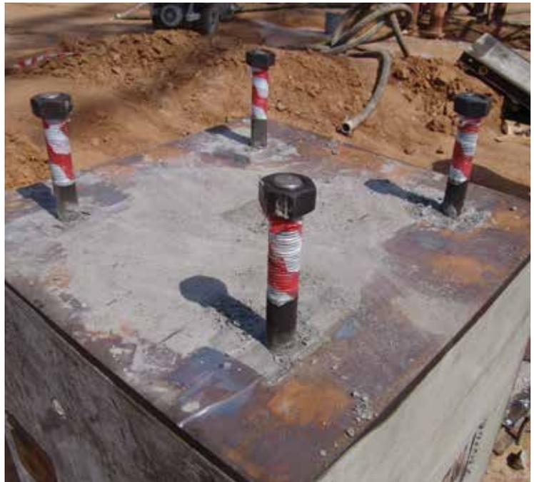
The use of anchor bolts for the column-to-column and column-to-footing connections was a departure from the normal Russian practice of welded connections in precast concrete construction. Bolted connections are commonly used in steel construction, however. *Courtesy of Building Design International.*
