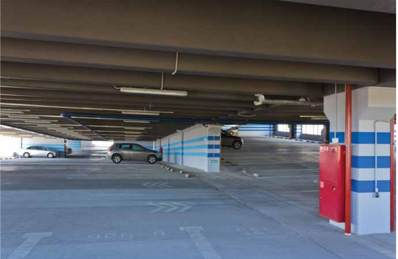
The structure has more walls than necessary to resist lateral forces due to the need for fire walls. **Courtesy of Building Design International.**
