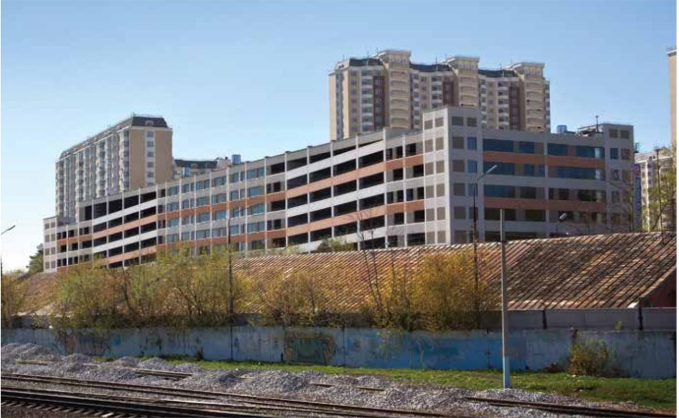
The parking structure at the Golovino residential complex in Moscow opened in March 2013. The local building code requires parking structures to be enclosed by glass on all sides within 50 m (160 ft) of residences (three sides in this case) to protect them from exposure to exhaust and fires. Sprinklers, ventilation, and a 90-minute fire rating are required in enclosed structures. *Courtesy of Building Design International.*
